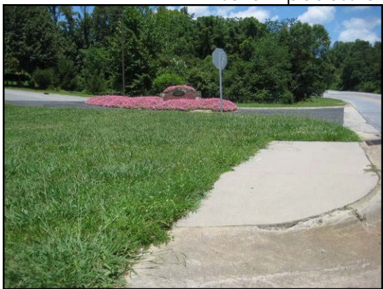
The sidewalk along Gridstaff Cove Road abruptly ends at the entrance to the Jackson County Justice & Administration Center, creating a barrier for pedestrian access to the public building.
