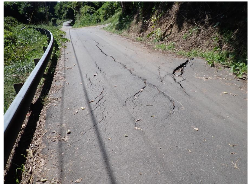
Figure 6A. Location A on map. Ground ruptures in Allen Street pavement. View looking SW. Inferred movement direction toward the SSW. 10/08/2020 NCGS photo.
