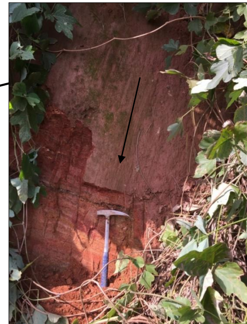
Figure 7B. Location B on map. Segment of the upper slide scarp (ground rupture) above Chipper Curve Road at location indicated in Fig. 7C. Arrow shows orientation of aligned grooves on scarp face from slide movement. Scraped section at hammer shows relict bedrock layering in completely decomposed biotite gneiss. Hammer handle is ~14in long. View looking NW. 10/08/2020 NCGS photo.
