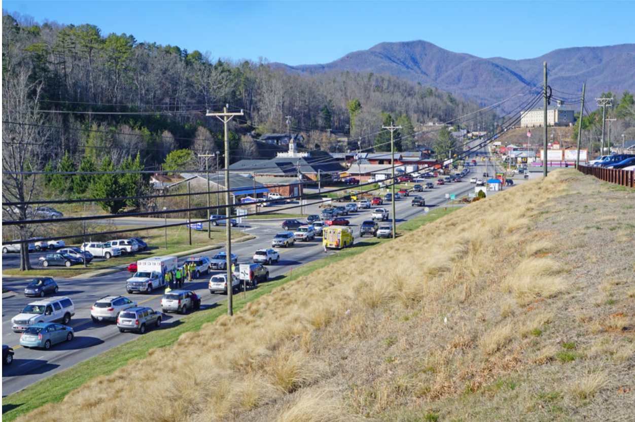
A high crash rate and congestion along NC 107 call for roadway changes. Image Source: The Sylva Herald.
