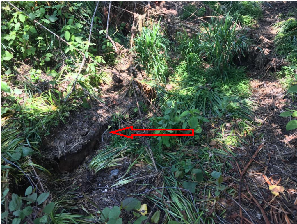
Photo 9: Tension crack observed within mid-slope bench, north end of failure. Photo dated 05/10/2020.
